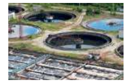
Aguas contaminada residuales Polluted water and waste water
